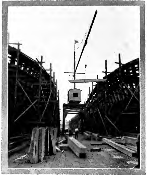
Shipyards designed and built by the Colby Engineering Company of Portland, Oregon. This crane is typical of the material handling rigs used in the wooden shipyards of the Northwest.
